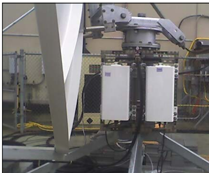
Antenna-mount 1:1 system w/ mounting frame
