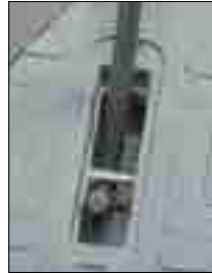
Recessed Lifting Pin with Cover
