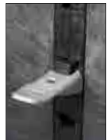
Step Bracket with Wedge
