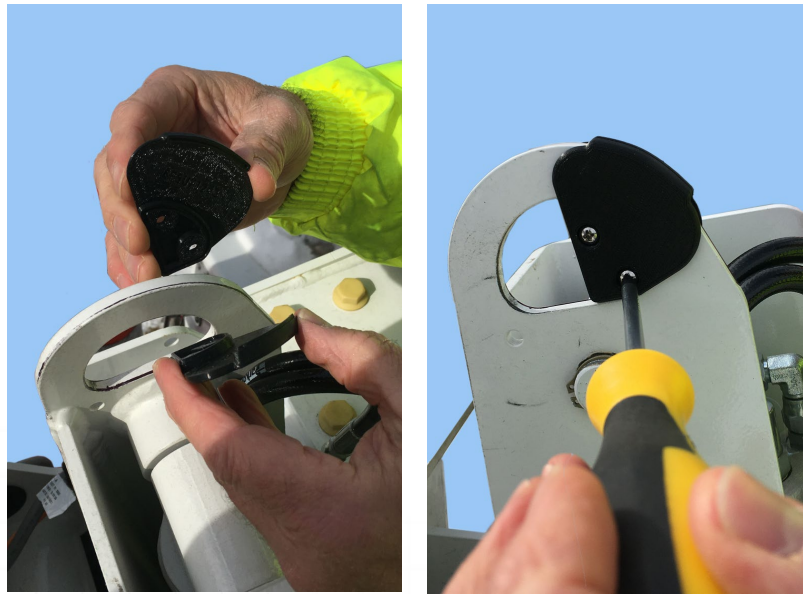
Figure 6: Installation of the SYS/4657 Anchor Block.
