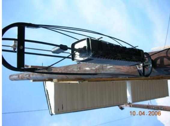
The fiber should already be placed flat on the ground for a distance, be dispensed from a reel, or entirely spread out for its full length. All fiber should be straight and flat, with *no twists*. The Opti-Loop Mini-Shoe does not introduce twist since the fiber drop is not “coiled”.
