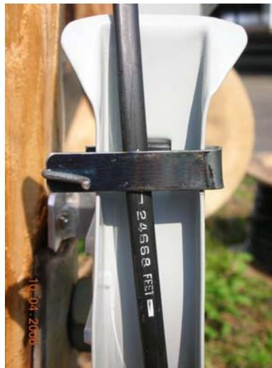
Place the fiber drop into the managing track by moving the locking latches (3) up away from their mooring and pushing the spring fingers far enough away from the device to permit the fiber drop to traverse into the track. *(This should only have to be moved approximately 5/16”.)*
