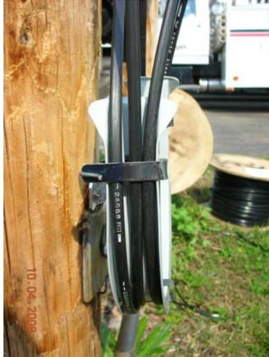
\*If the drop is being placed in conduit or direct breeied, then follow the path and procedure around the upper Opti-Loop Mini-Shoe, then to the conduit or into the earth.
