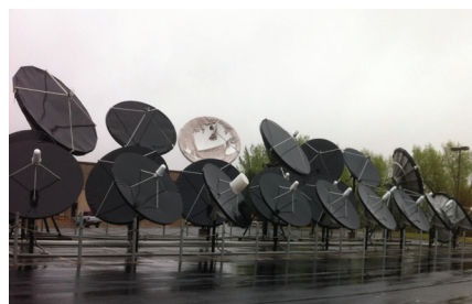
Ground Mounted Antenna Farm
