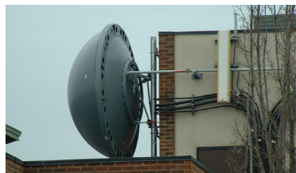
Microwave Antenna Installation
