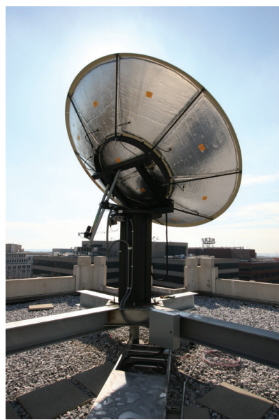
3.8M Antenna with Full De-Icing System Installed
