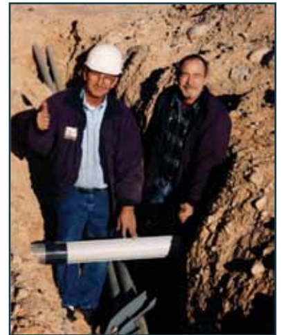
5 – Job Finished in Record Time
