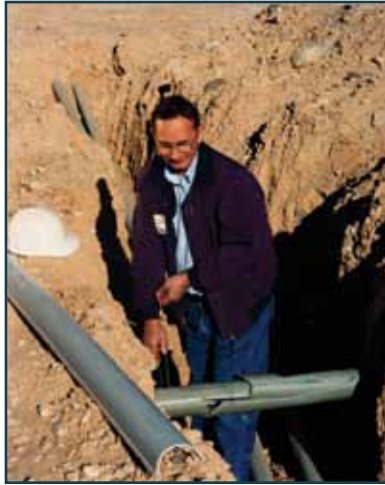
1 – Remove Damaged Conduit
