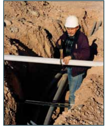
2 – Cut Split Duct to Length
