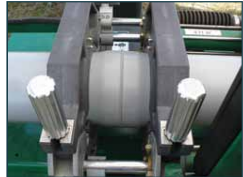
Pipe ends are held under pressure until newly-formed joint cools.
